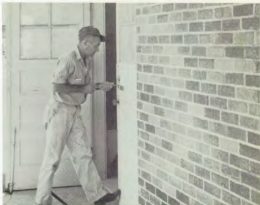
Frank Cobos busily makes repairs about the school.
